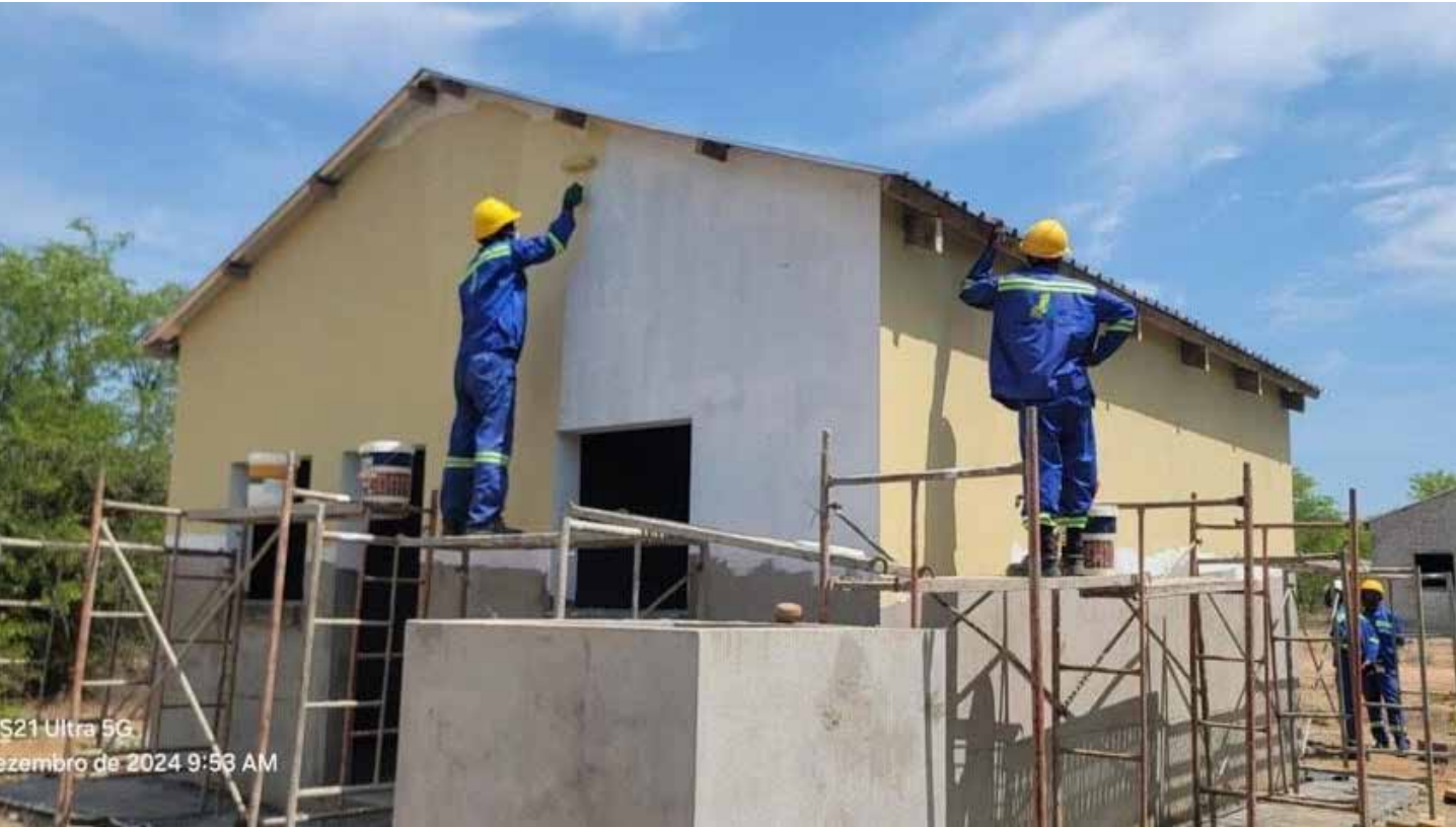
Construction of Mavodze's resettlement houses at Macuacane site
