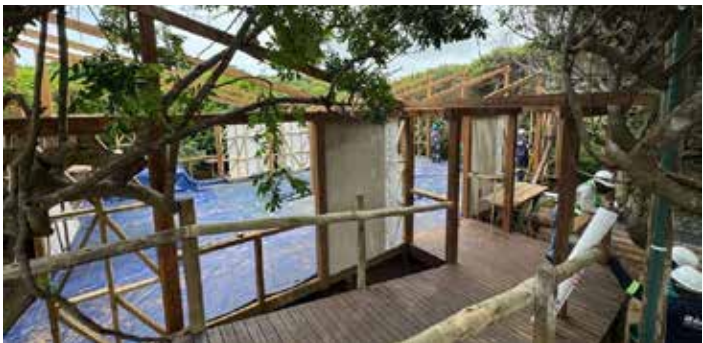
The Conference Center construction had progressed to schedule and will be opened in May 2025- boosting park mid week tourism activities and occupancies.
