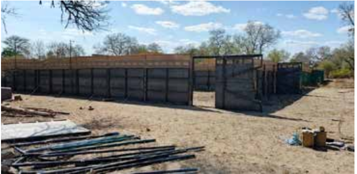
The park constructed four additional steel bomas and are ready to receive the planned additional ten black rhino in 2025
