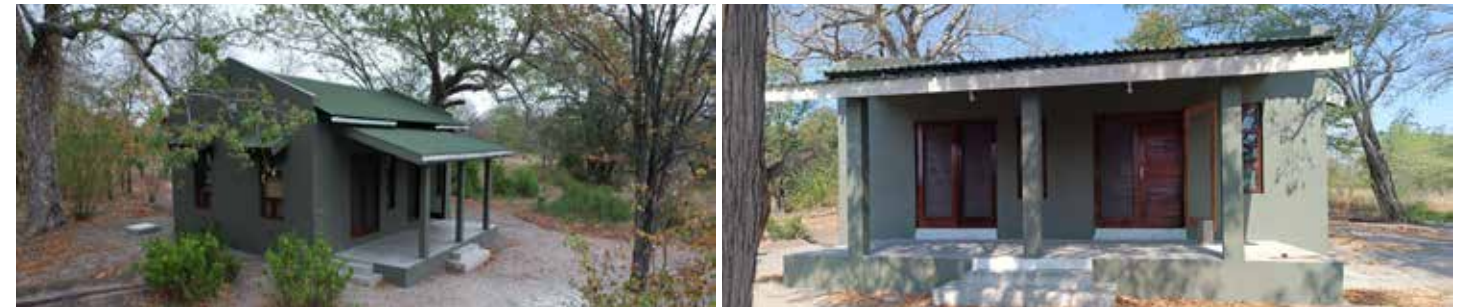
The construction of new staff housing, managed by the park, is a milestone to improving living and working conditions in this remote park
